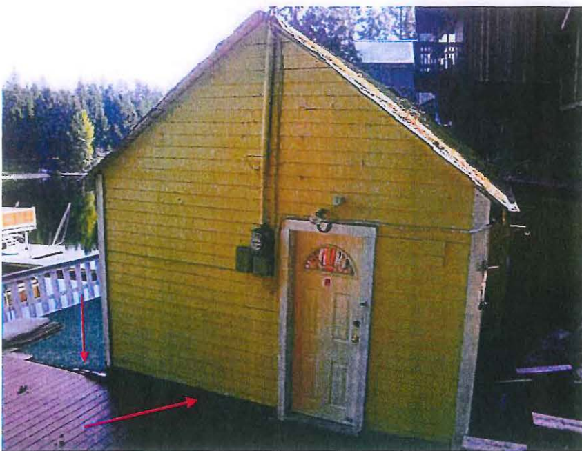
Photo 2. The western side of the cabin. Note the areas marked with red arrows, as they indicate zones of structural instability for the deck and cabin.
