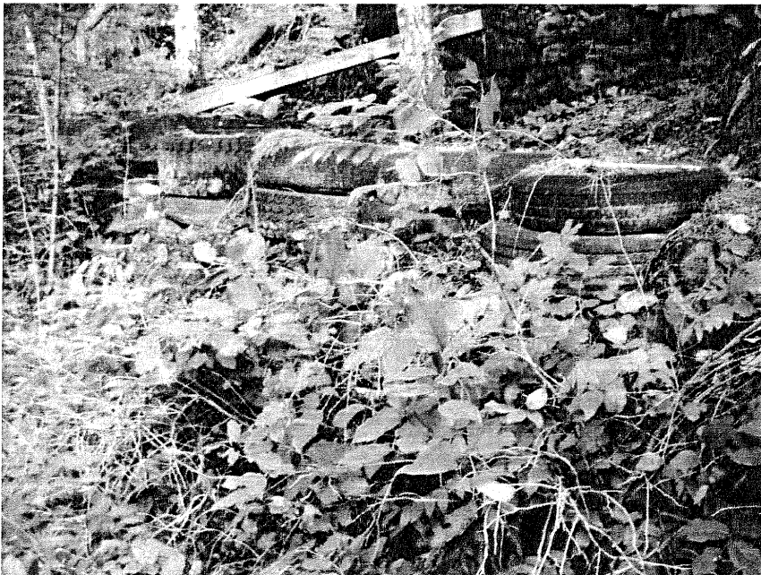
Photo 7: Looking northwest at the upper portion of the switchback trail and slope, both of which are in the SPEA. Note the old tires that are being used to reinforce the stability of the bank.
