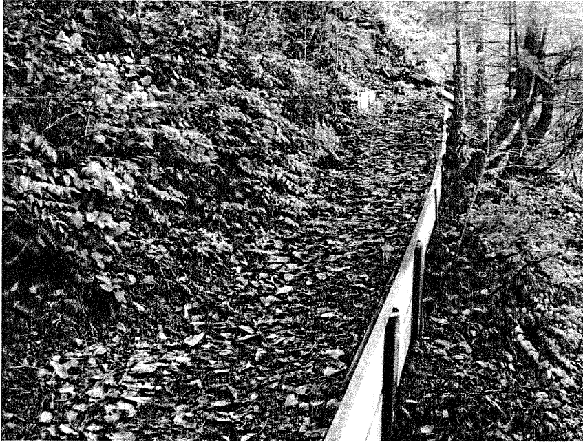
Photo 6: Looking east at a middle portion of the switchback trail that is located within the SPEA. Note the 2"x12" boards that are used to reinforce the trail.
