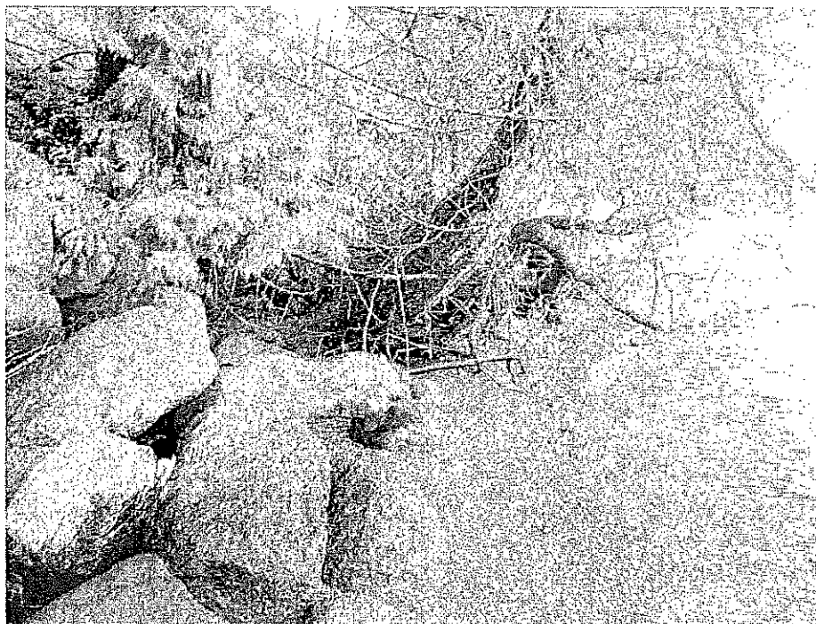
Photo 4 – Failed shoreline protection near toe of slide area looking westward
