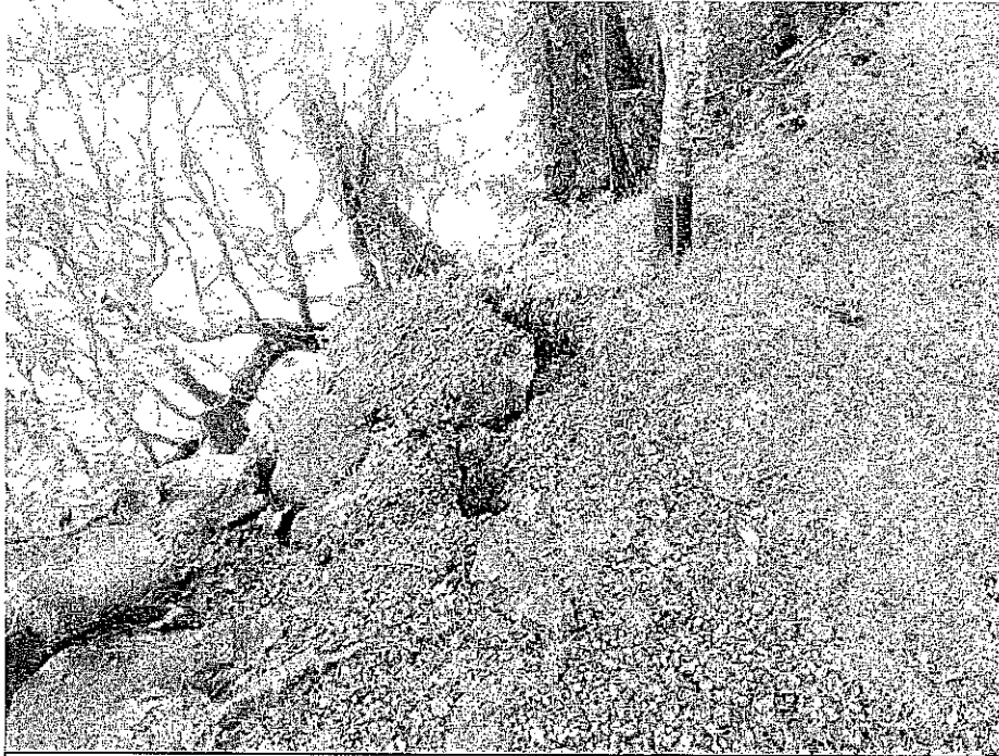
Photo 5 – Tension cracks near crest of slope above failed shoreline protection
