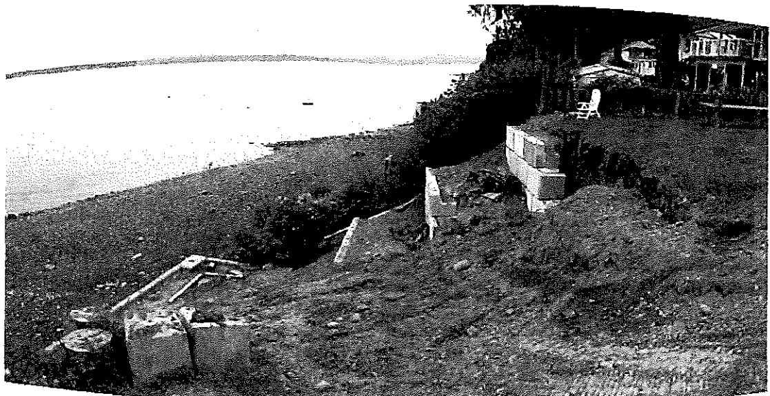
View of the project location. The three Lock-Block retaining walls are under construction, visible within the centre-right portion of the photo.
