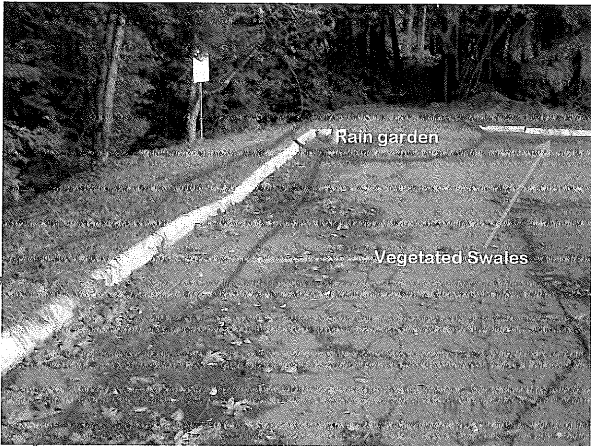
Photograph 2. Part of the Kerry Park Arena parking lot drains directly to Shawnigan Creek. Construction of vegetated swales leading to a rain garden would be a simple way of treating parking lot drainage.
