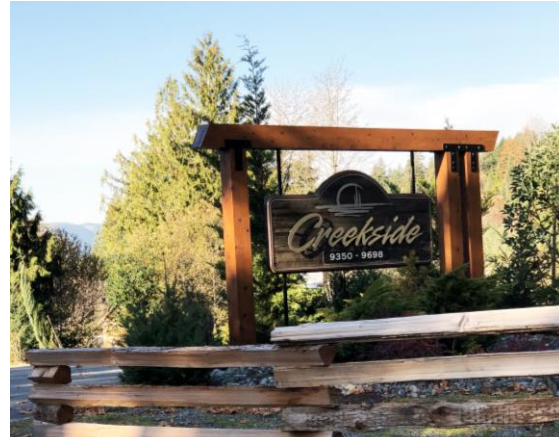
Image 23: Free standing signs should carry a low profile, framed with heavy timber.
