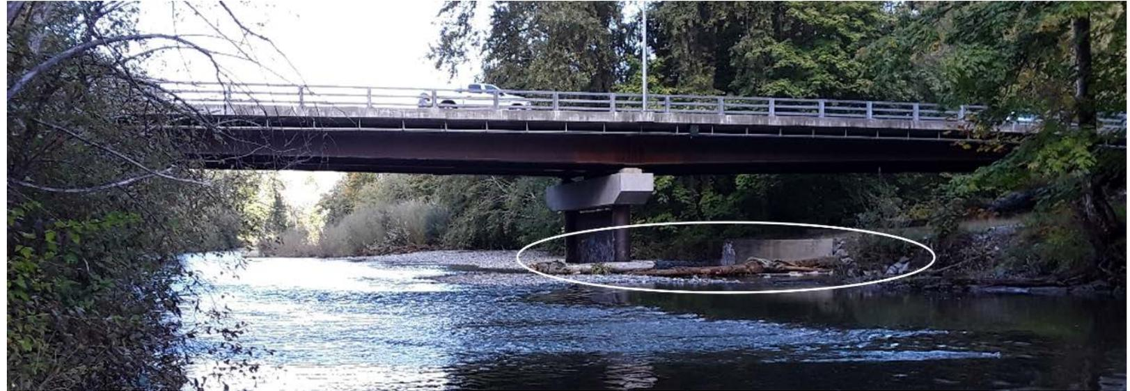
▲ Photo 3.3 Multiple logs, floated downstream by a 2021 flood, caught on the foundation structures of the Highway 1A bridge.
