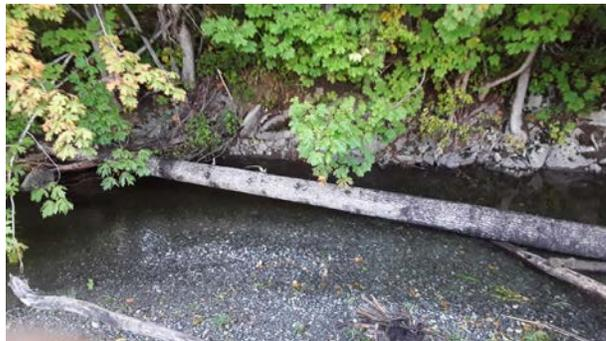
◀ Photo 3.2 Back-channel bank is armoured by riprap, which shows signs of scour along the toe.
