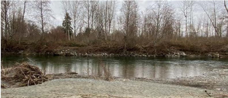
▲ Photo 2.5 The bar tail has a high proportion of sand. The bank opposite the bar has been stabilized with riprap.
