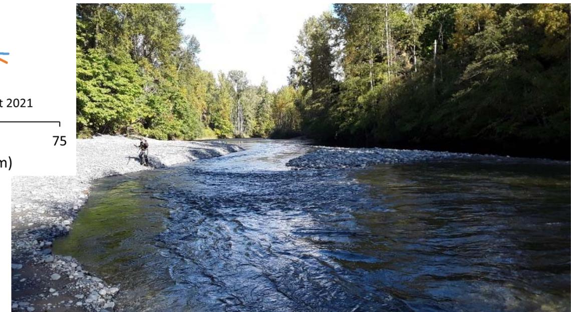
► Photo 5.13 Sediment was removed from the bar tail (2021) to create a wider wetted channel and to reduce flow towards the opposite bank.
