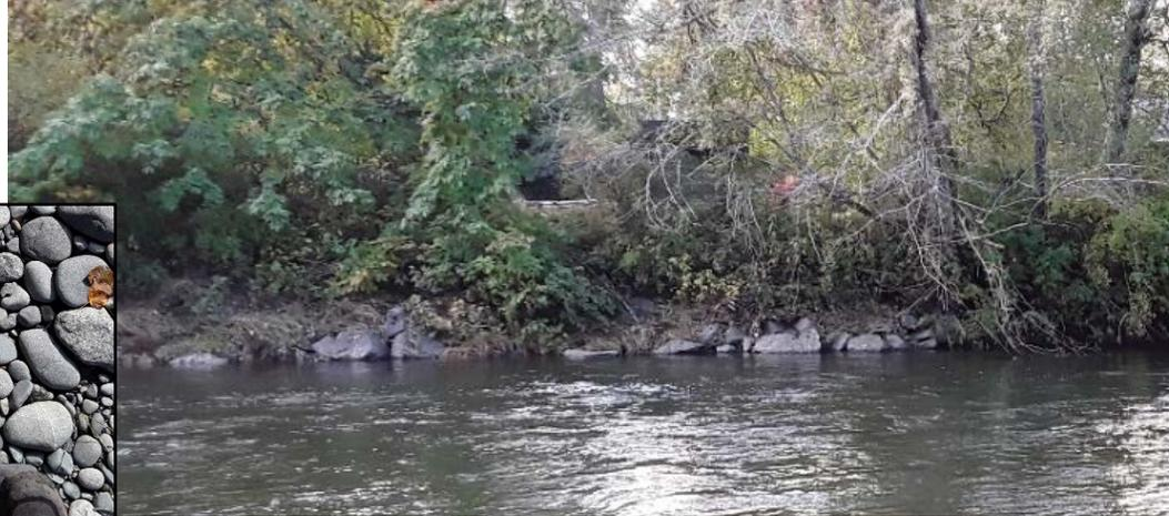
► Photo 2.3 Downstream of the riprap, the bank is composed of silty material with clay and fine sand. The toe of the bank is a gravel-sand mix.
