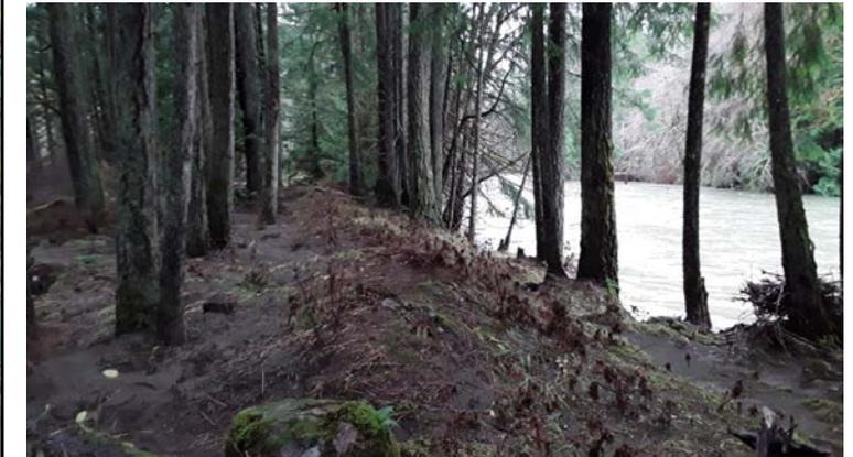
▲ Photo 6.3 Earthen berm reduces the amount of flow that spills out onto the floodplain during peak flood events.
