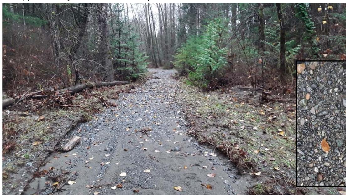
► Bed lowering along the left side of the channel at RK 5.8, resulting from sediment removal in 2021.
