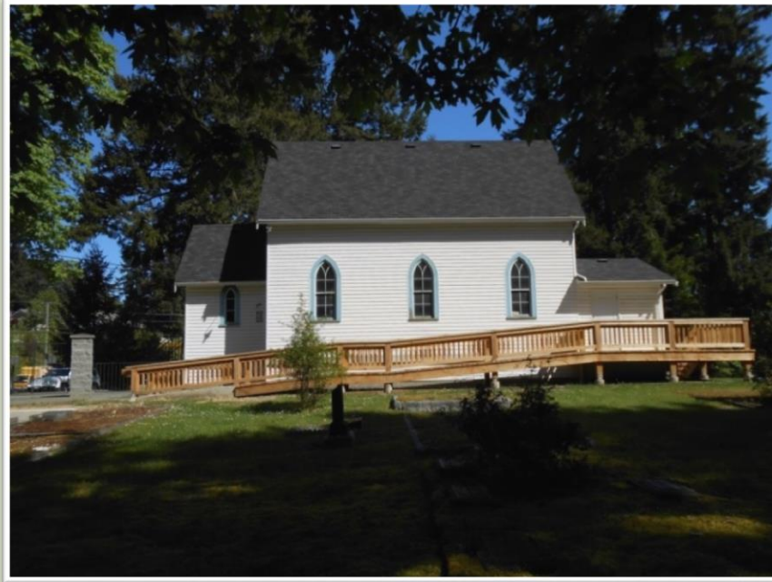
View of the new wheelchair accessible ramp
