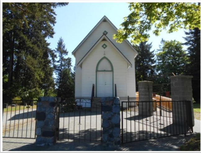
Front View of Church
