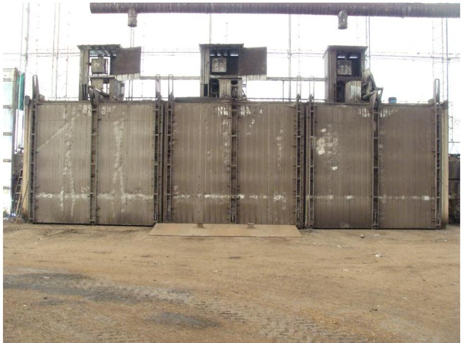
Excess exhaust air from the in-vessel composting boxes is ventilated through a biofilter, as is the 30,000 cubic ft of air from the receiving, mixing and curing building.
