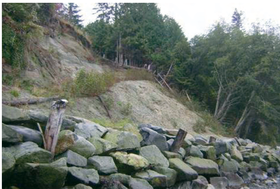
FIGURE 2.10: Example of a hardened shoreline
