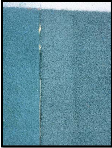
TURF SEAM SPLITTING
