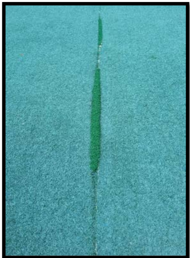
PATCHED TURF SEAM
