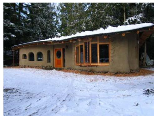
***OUR Ecovillage's demonstration building features cob construction, a green roof and an earthen floor.***
