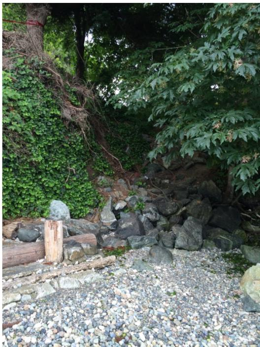
Photo 10. Remnants of rock armouring at the road right-of-way and exposed tree roots from erosion.
