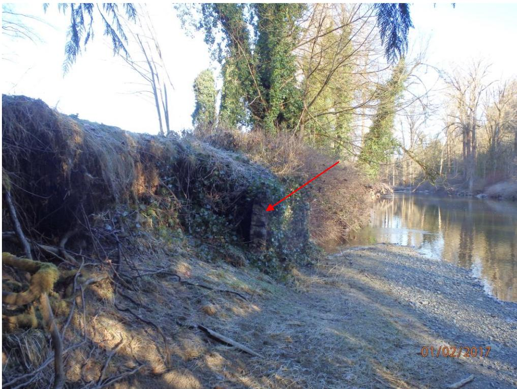
Remains of concrete retaining wall (highlighted) and localized erosion of the bank along the edge of the lawn area.
