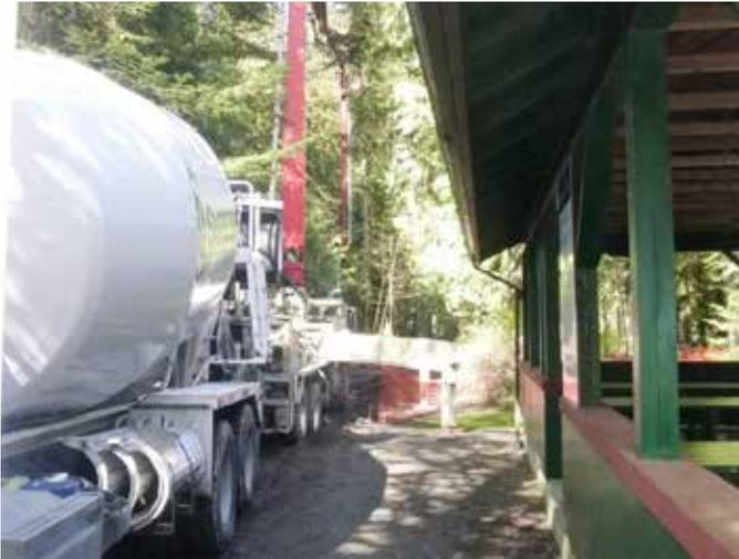
Concrete and pumper truck placing concrete at outdoor classroom/ amphitheatre
