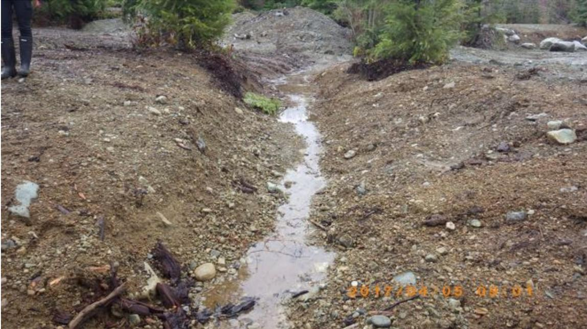
Figure 38. A second drainage channel leads surface flows across the recent man-made terrace, discharging into the soils at the top-of-slope, as shown in Figure 37.
