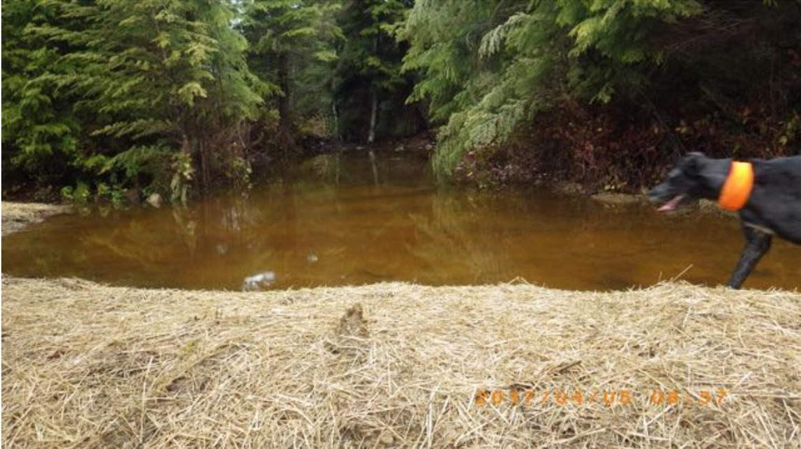
Figure 34. Looking across the newly constructed berm that prevents the wetland flows from being routed down the driveway drainage channel. The wetland extends north along the axis shown in the photograph approximately 100 metres. This wetland is fed by springs and seepage from the slope to the east.
