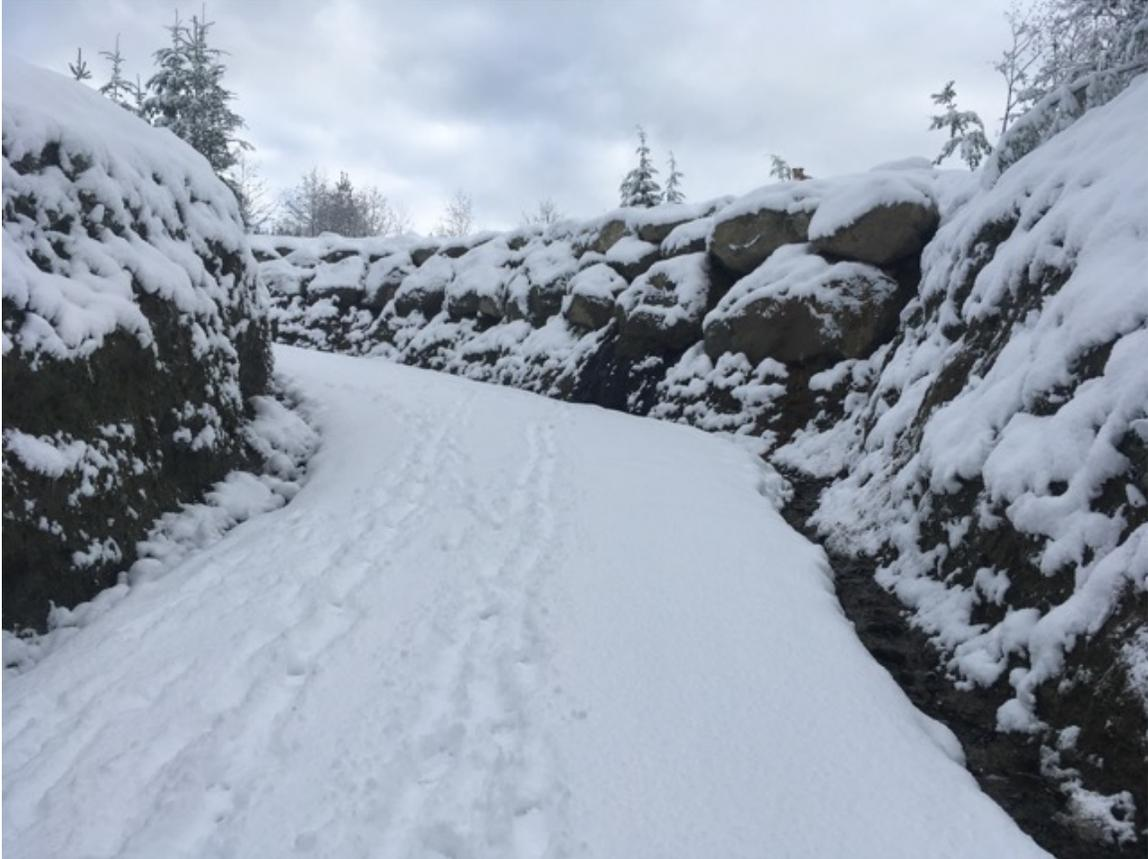
Figure 31. Looking east up the driveway, showing the initial rock stack wall. The boulder wall will be removed and a terrace constructed to reduce the vertical height of the wall.
