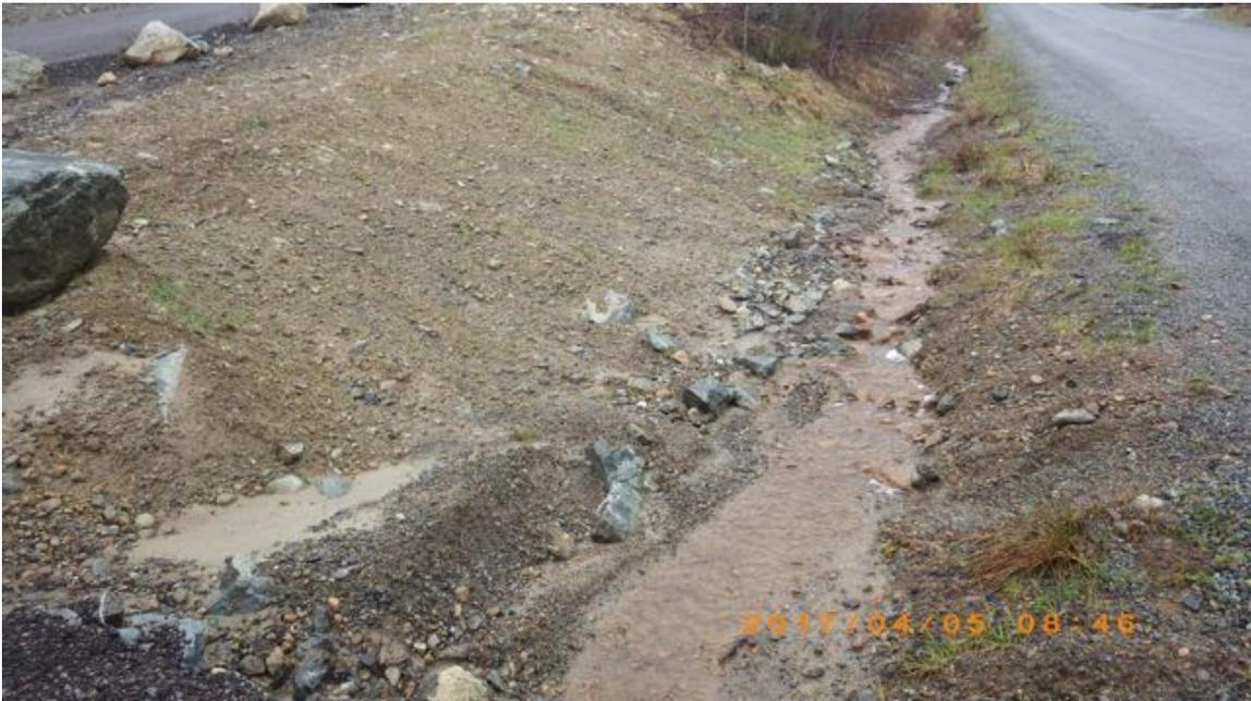
Figure 26. Drainage in the road side channel is largely from the drainage flowing on the south side of the driveway access (Figure 27).
