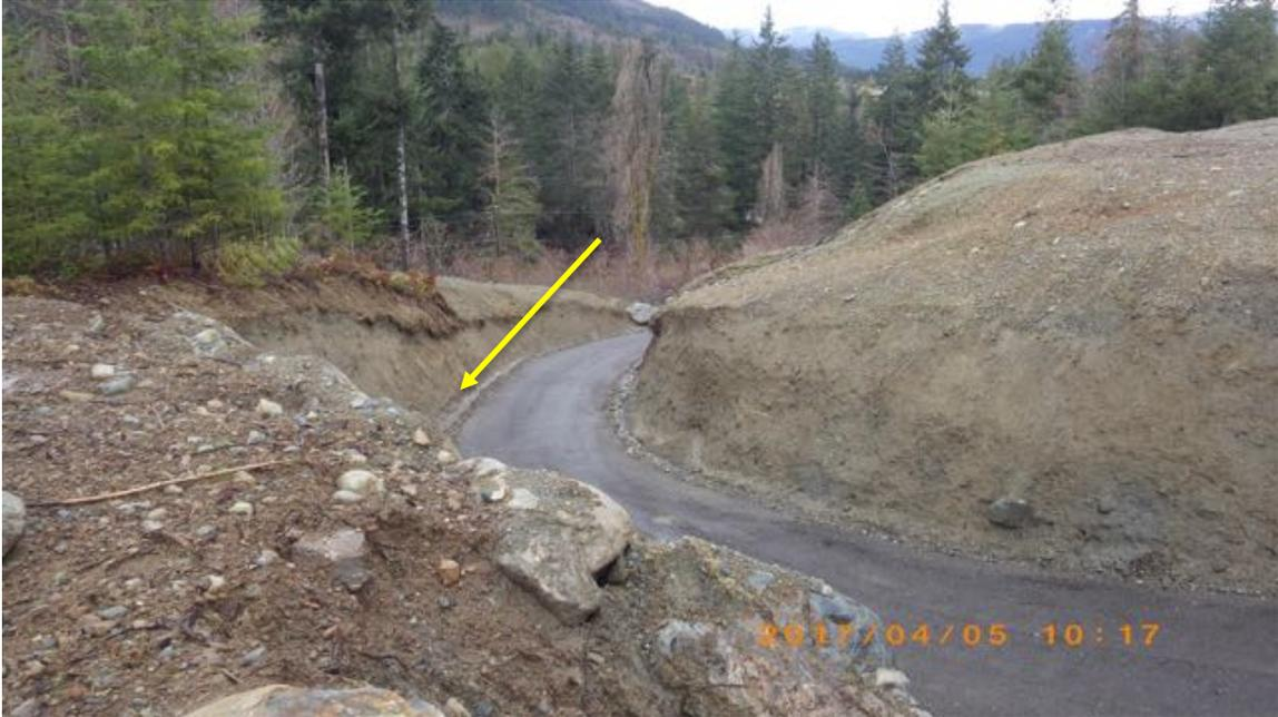
Figure 29. North Lot, looking west and downslope at the driveway access road leading from Stebbings Road upslope to the building site. The drainage channel lies on the south side of the driveway (yellow arrow).
