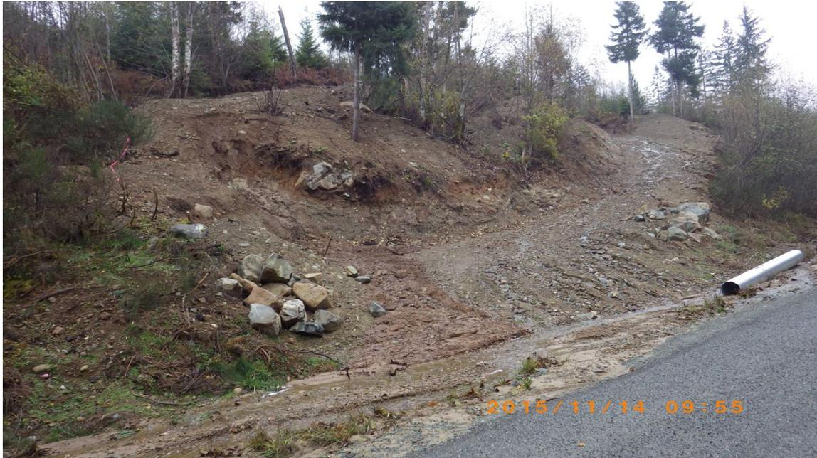
Figure 19. Looking east across the newly, partially constructed driveway access leading to the proposed building site on the terrace. Note the sediment in the road side drainage channel; the sediment is primarily from disturbed soils associated with the driveway construction. Contrast this image with that in Figure 20.
