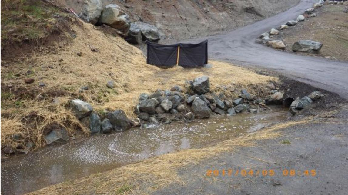
Figure 23. Runoff entering the road side drainage channel is carrying sediment and has a low level of turbidity.
