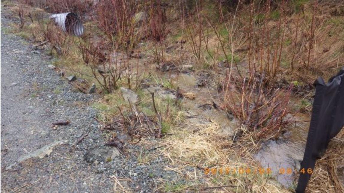
Figure 25. The road side drainage channel discharges into a CSP culvert under Stebbings Road. Note the turbid flow and sediment trapped within the vegetation.
