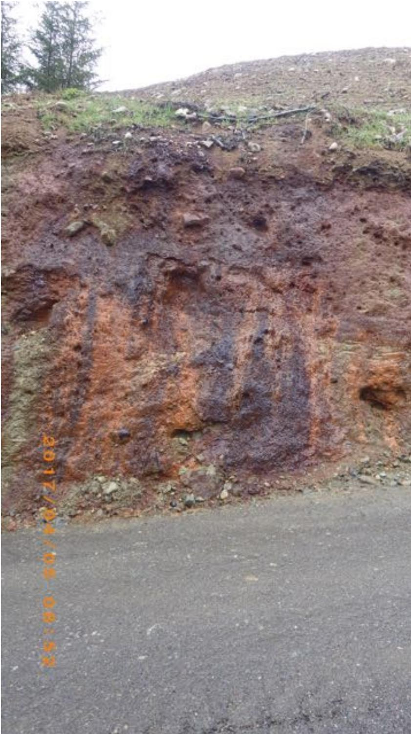
Figure 33. Vertical wall, consisting of compacted glacial till, showing ground water seepage. The rust stain consists of iron bacteria.
