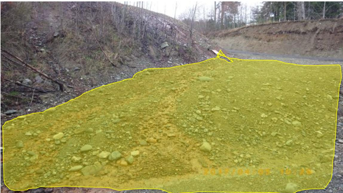
Figure 18. The yellow polygon must be planted with grass seed and covered with wood chips.
