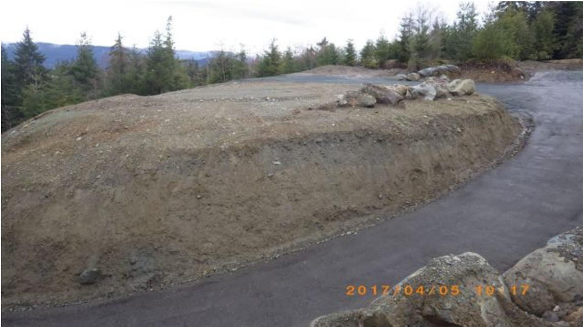
Figure 30. North Lot, looking northwest across the driveway access road to the proposed building site. The steep slope will be terraced to reduce the vertical wall height.
