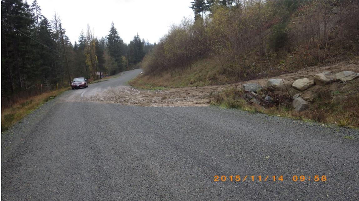
Figure 15. Sediment flowing across Stebbings Road following a moderate rain storm.
