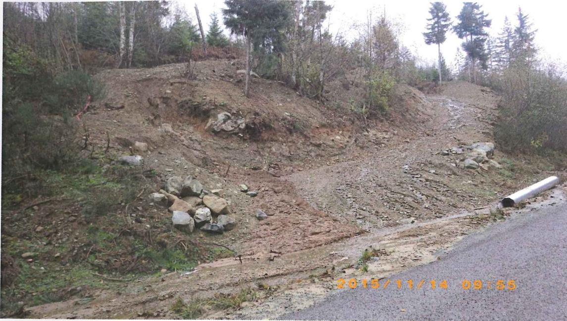
Figure 19. Looking east across the newly, partially constructed driveway access leading to the proposed building site on the terrace. Note the sediment in the road side drainage channel; the sediment is primarily from disturbed soils associated with the driveway construction. Contrast this image with that in Figure 20.
