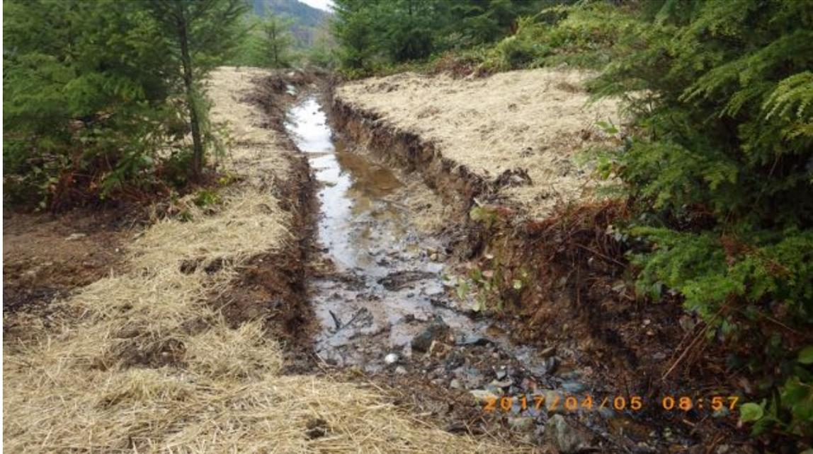
Figure 36. Looking west at the drainage channel routing wetland overflows to the bank adjacent to Stebbings Road.
