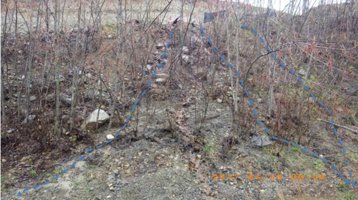
Figure 27. Runoff from the driveway access road flows across the steep slope into the road side drainage on Stebbings Road.
