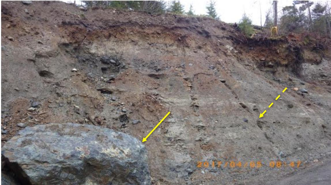
Figure 21. A close up of the glacial till bank. The rock (yellow arrow) can be seen in Figure 22. Note the erosion of the bank material. This bank will be reshaped to eliminate the steep vertical face, in the late summer of 2017. The dashed arrow identifies an erosion rivulet seen in an oblique angle in Figure 22.
