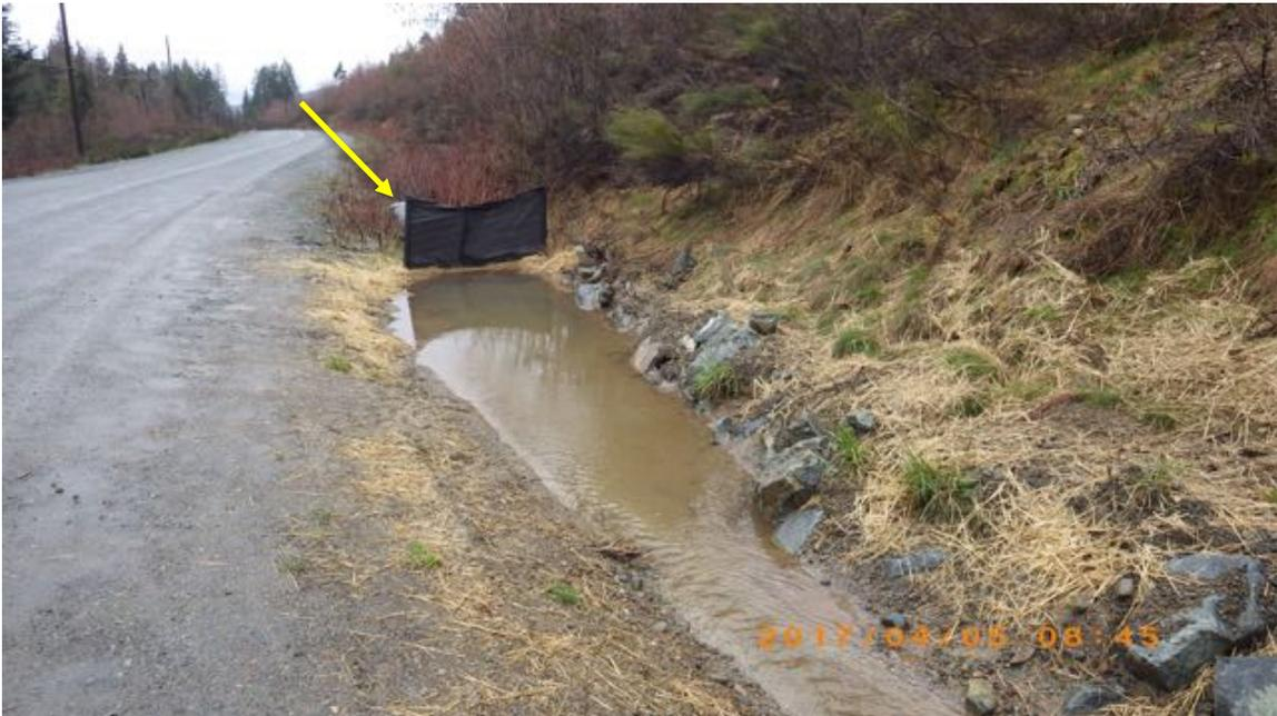
Figure 24. Looking north along Stebbings Road. The road side drainage channel discharges into a culvert under the road (yellow arrow) (Figure 25).
