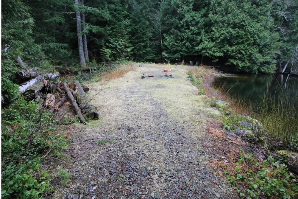
Photo 11 Dam crest wider than design drawings
