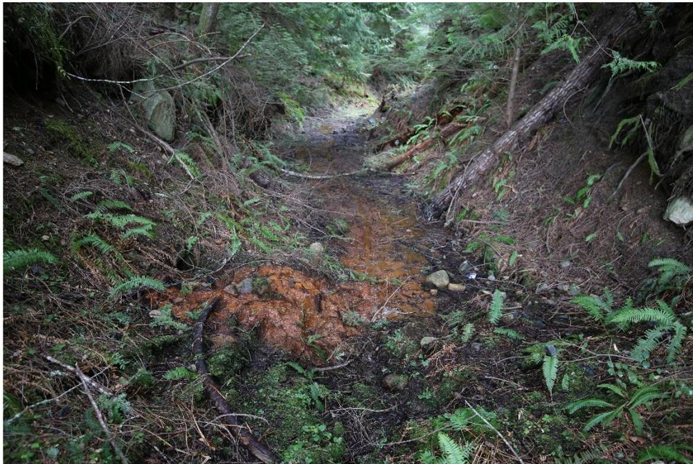
**Photo 10** Backfilled water main trench downstream of the dam, note saturated surface
