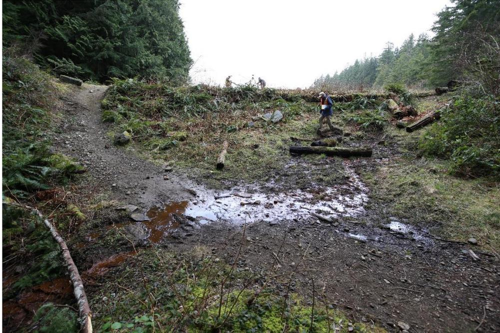
**Photo 3** Seepage located at the left abutment toe, March 29, 2018
